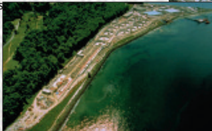
Water and Waste Water Treatment Plants
